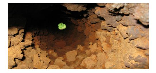
This photo is from the inside of an old cast iron water main that was replaced in 2011 which had been in service since 1931. Looks like the inside of a cave! The Louisville Water Company used the pipe bursting method which is trenchless and can utilize the existing easements/right of way. Don't worry. Your water mains are most likely of the newer variety. Photo from Wayne Kimbel
